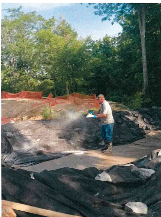
June 22 - Manhole 1750 During Cleanup
