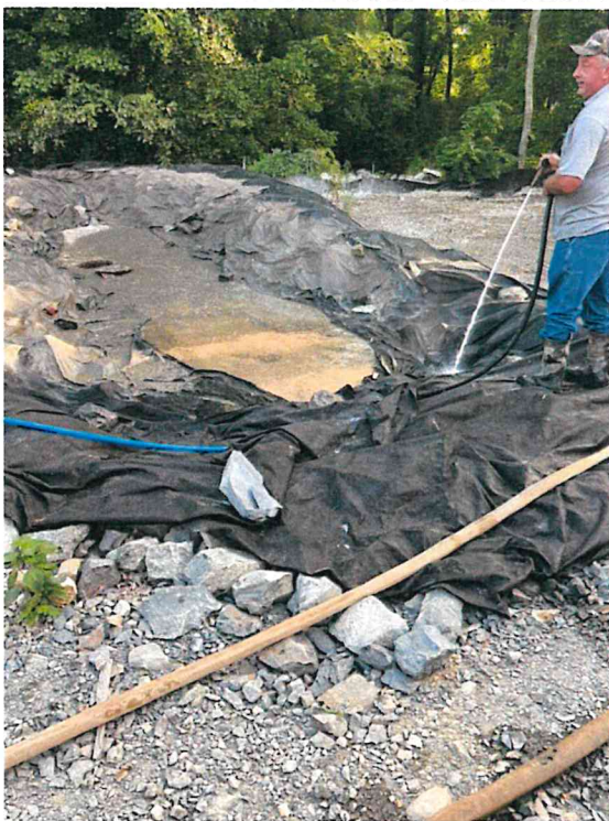
June 22 - Manhole 1750 During Cleanup
