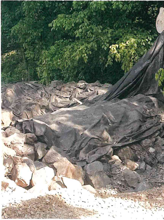
June 11 - Manhole 1750 During cleanup
