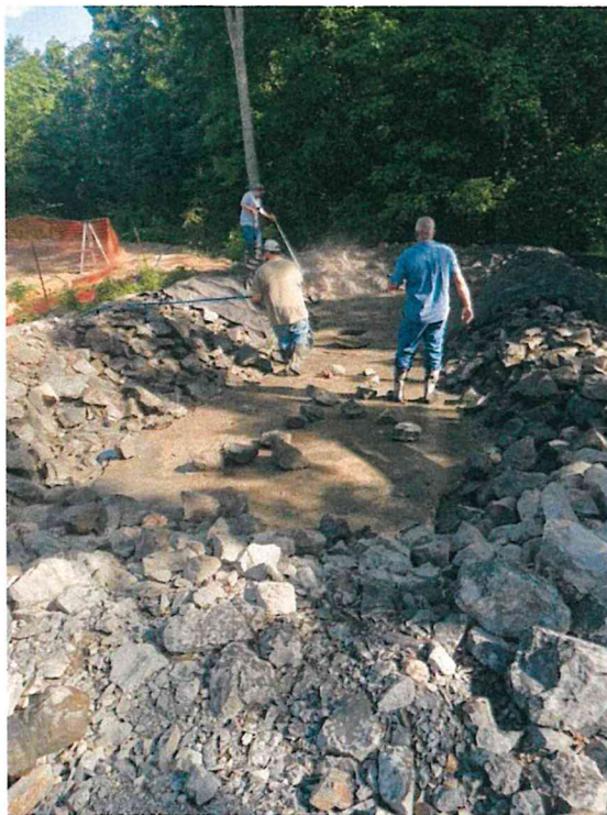
June 11 - Manhole 1750 During cleanup
