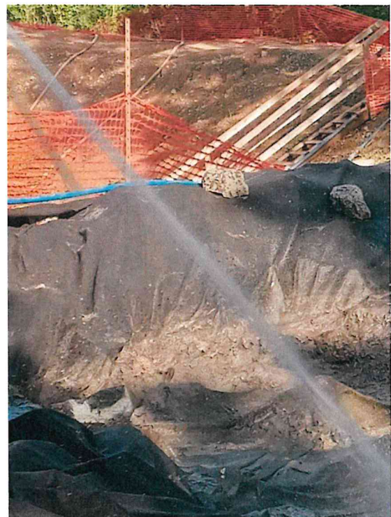
June 11 - Manhole 1750 During cleanup
