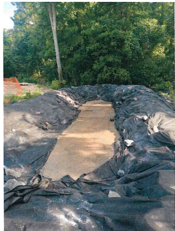
June 22 - Manhole 1750 After cleanup
