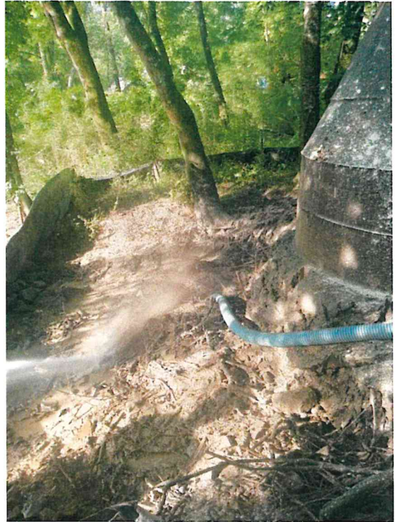
June 11 - Manhole 1748 During cleanup
