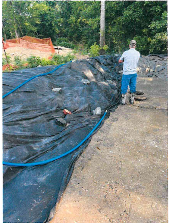
June 22 - Manhole 1750 During Cleanup
