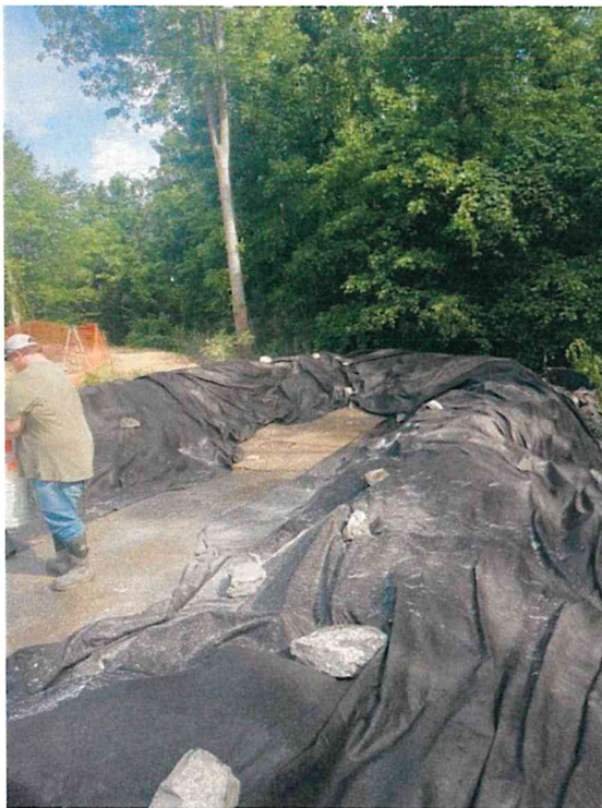
June 11 - Manhole 1750 During cleanup
