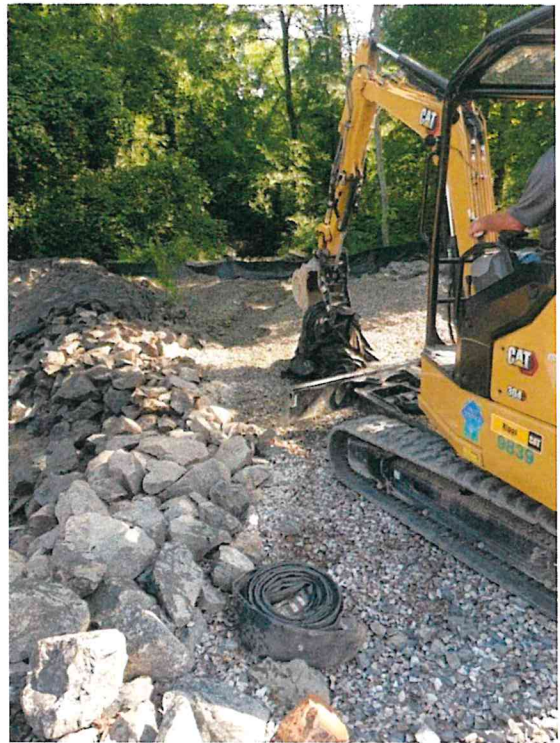
June 11 - Manhole 1750 During cleanup
