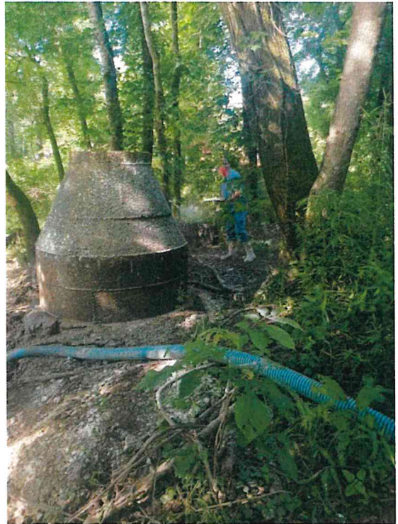
June 11 - Manhole 1748 During cleanup
