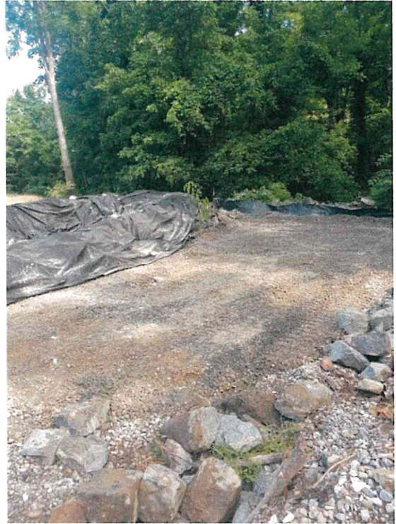
June 11 - Manhole 1750 After cleanup
