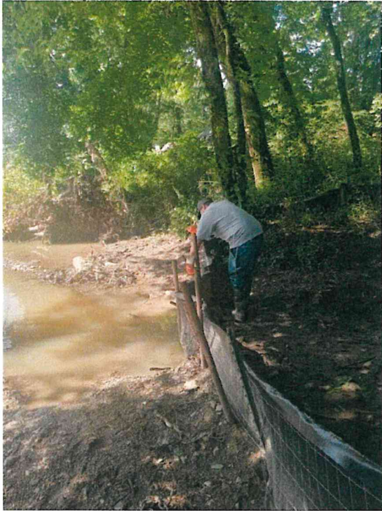
June 11 - Manhole 1748 During cleanup
