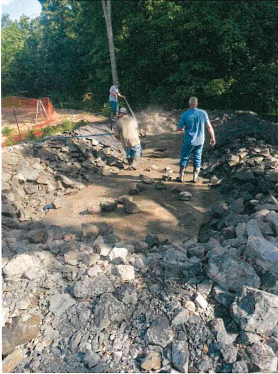
June 11 - Manhole 1750 During cleanup
