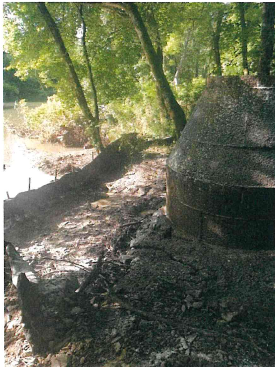
June 11 - Manhole 1748 After cleanup
