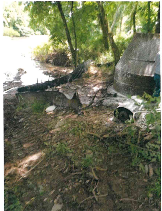
June 11 - Manhole 1748 During cleanup
