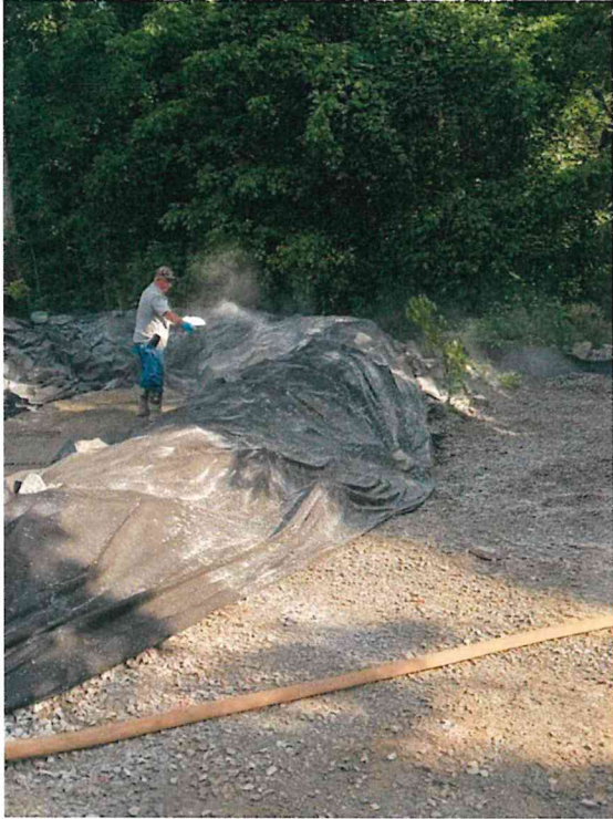
June 22 - Manhole 1750 During Cleanup
