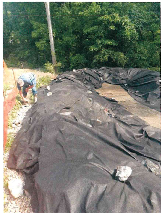
June 11 - Manhole 1750 During cleanup
