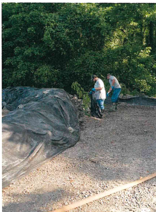
June 22 - Manhole 1750 During Cleanup
