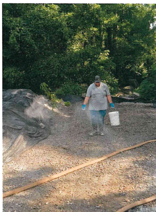
June 22 - Manhole 1750 During Cleanup
