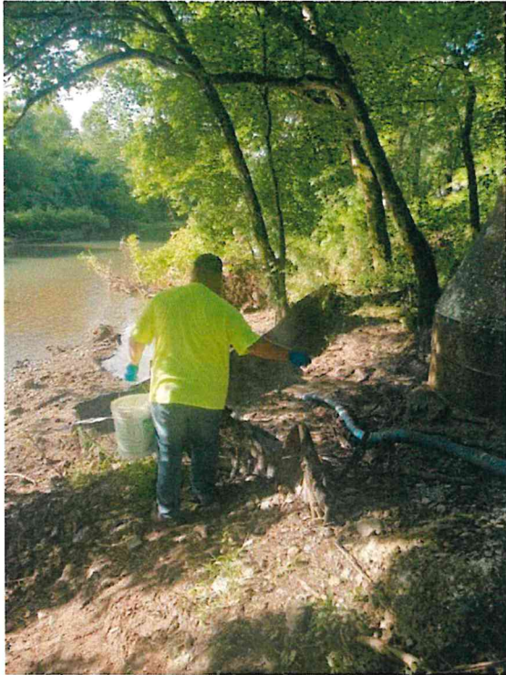
June 11 - Manhole 1748 During cleanup
