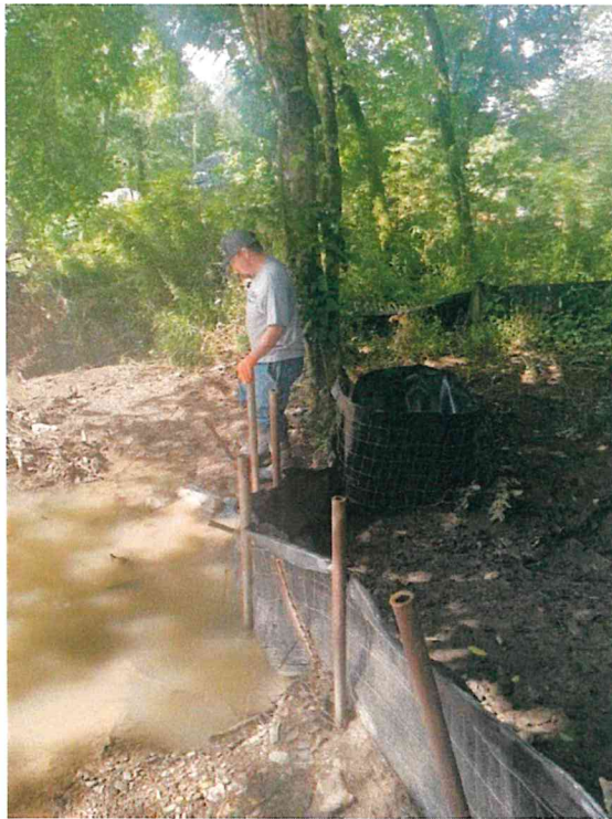
June 11 - Manhole 1748 During cleanup
