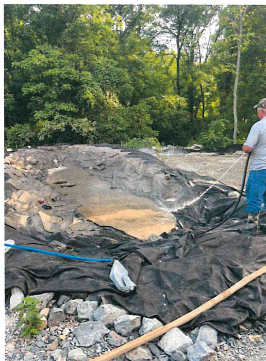
June 22 - Manhole 1750 During Cleanup
