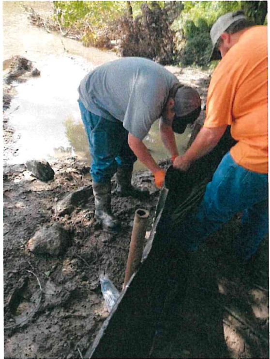
June 11 - Manhole 1748 During cleanup
