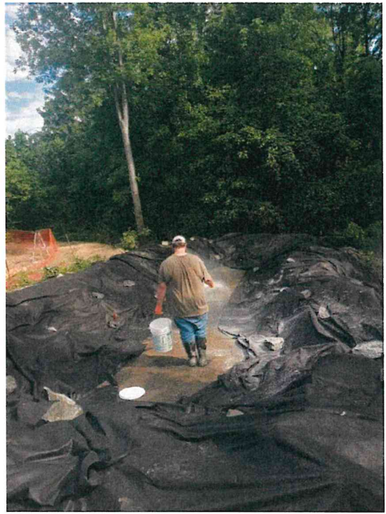
June 11 - Manhole 1750 During cleanup
