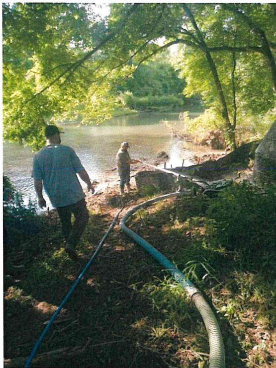
June 11 - Manhole 1748 During cleanup
