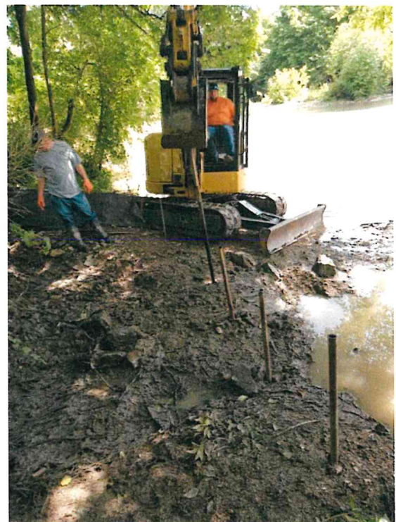
June 11 - Manhole 1748 During cleanup
