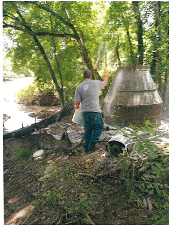
June 11 - Manhole 1748 During cleanup
